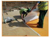
Step 3. Working in pairs, roll out the mat progressively whilst peeling away the release paper. For large areas, use a dry roller to smooth out.
